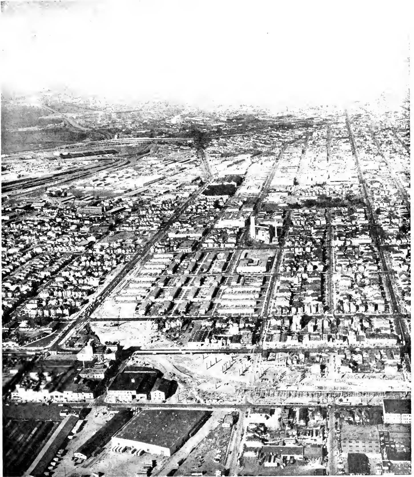
Construction scene on Eastshore Freeway project in Oakland from Market to 10th Street where route turns into Cypress Street and runs north. The 1.4-mile section along Cypress from this project to the distribution structure is scheduled to be started this year as a two-level viaduct at an estimated cost of $7,015,000.
